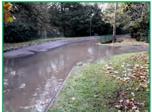
Flooding this winter on Church Lane
